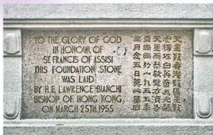
The foundation plaque at the right hand side of the Church's main entrance.
