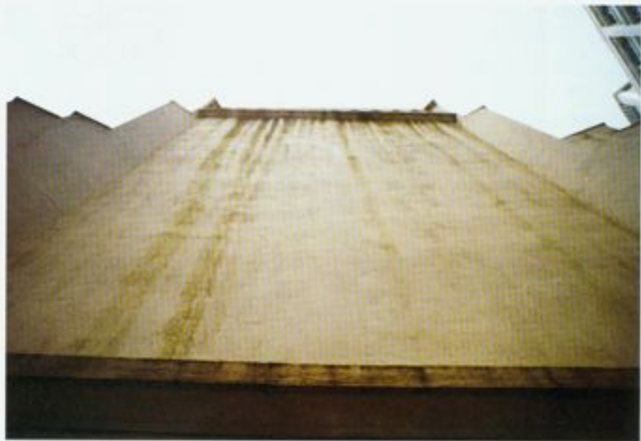
外壁 - an outside wall
