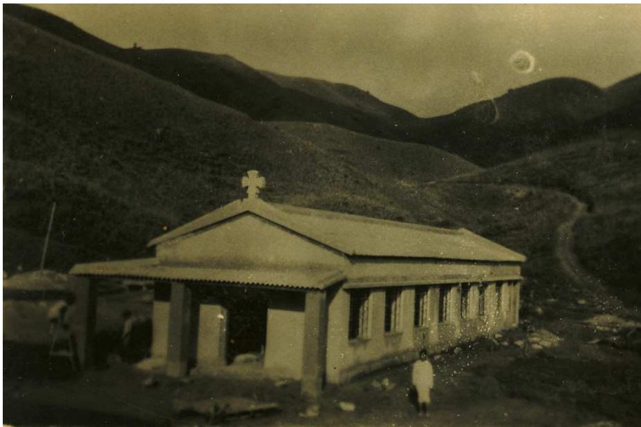
圖片(26)：這是興建神樂院時，修士們的臨時宿舍。 This was the temporary dormitory of the Trappists during the building of the Monastery.
