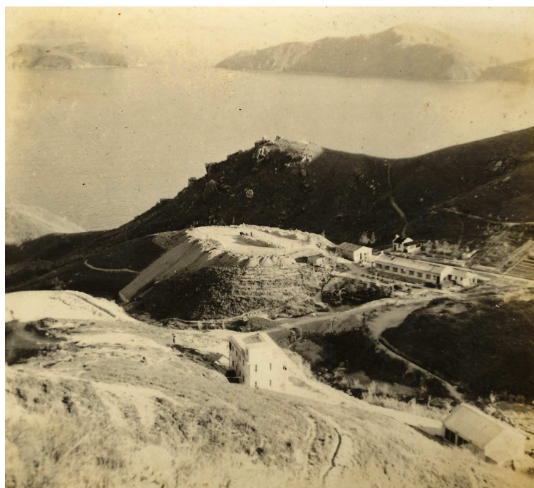
圖片(30)：從上俯望神樂院地盤。 A look of the site of the Monastery from above.
