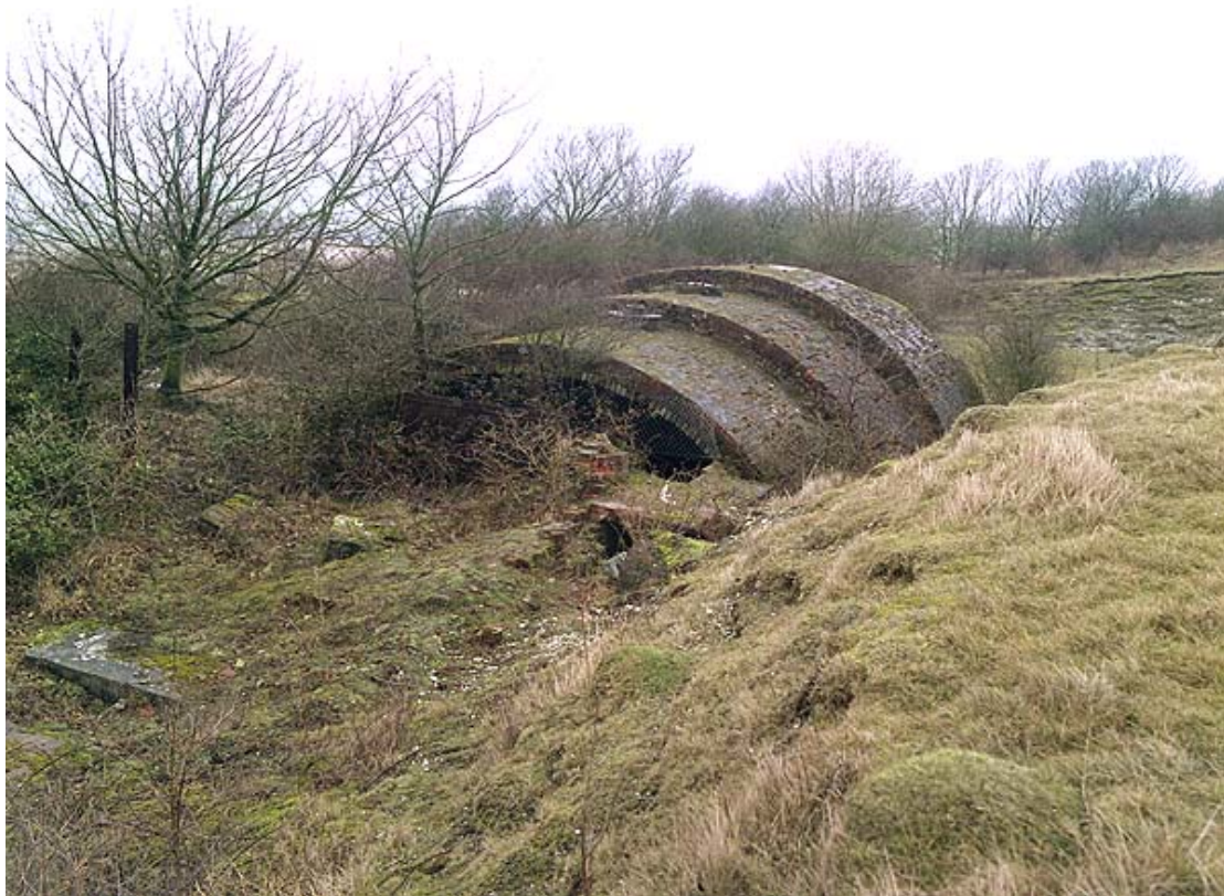
Experimental Shaft Kiln, Beddingham, East Sussex, used as a continuous mixed feed lime kiln in 1931-32.
