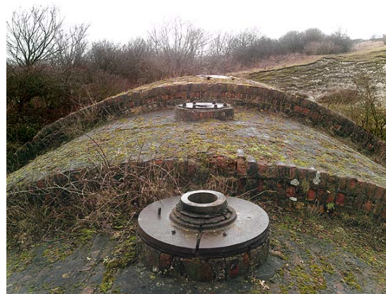
Circular steel plates on top of the barrel vaults
