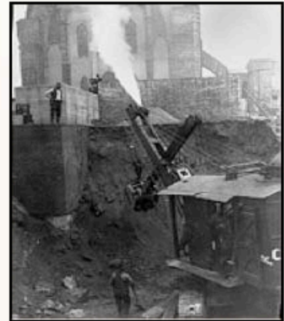
Digging the Cathedral's foundation
