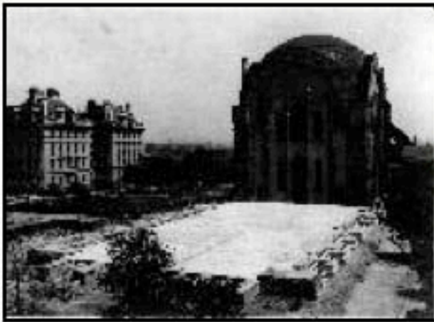
The foundation of the nave
