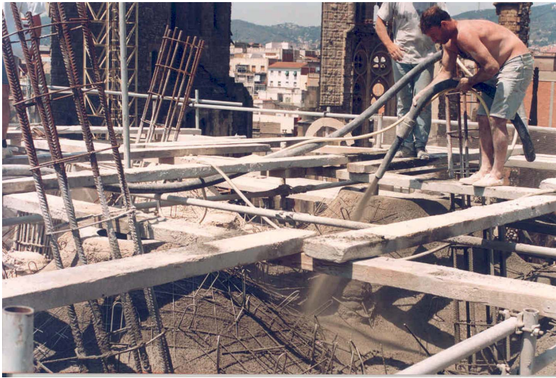
Figure 7. Photograph of concrete spraying (figure is provided in color online).
