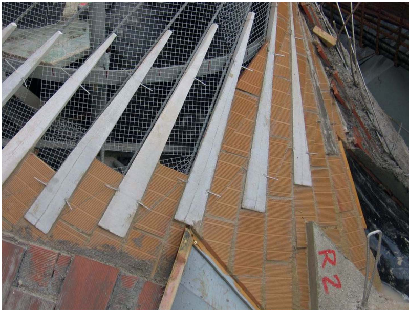
Figure 11. Photograph of the details of the first layer of tiles (figure is provided in color online).
