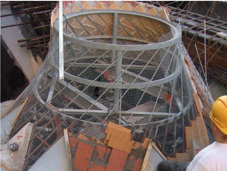
Figure 13. Photograph of the details of the first layer of tiles (figure is provided in color online).
