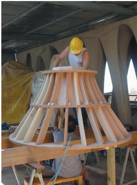
Figure 19. Photographs showing the formwork of the hyperboloids when they are placed on the superior part of the capital (figure is provided in color online).
