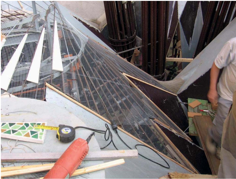
Figure 10. Photograph of the preparation of the hyperboloids (figure is provided in color online).
