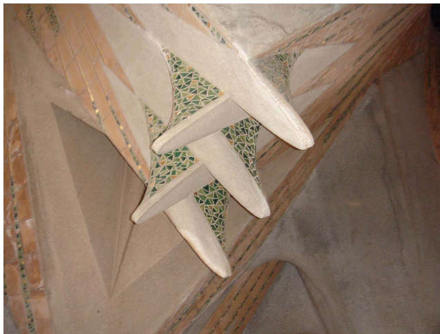
Figure 5. Photograph of detail of an intersection between hyperboloids and paraboloids (figure is provided in color online).
