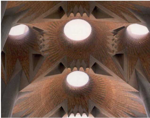
Figure 4. Photograph of the intersection between hyperboloids and paraboloids (figure is provided in color online).
