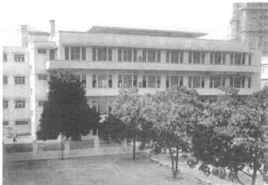
The old Orphanage demolished in 1983.
