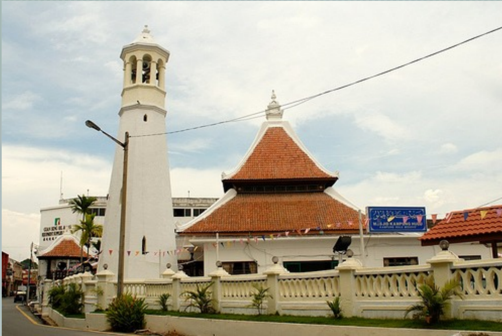
Kampung Hulu Mosque, built in 1728
